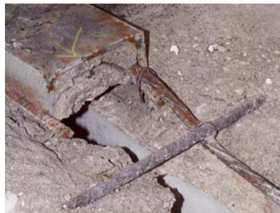
Prestressing strand in anchorage zone
