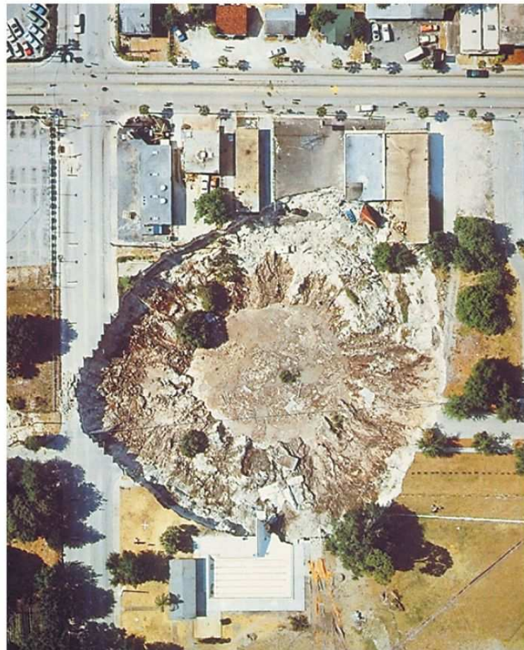
Figure 3. Winter Park, Florida. A number of massive sinkholes appeared here within a matter of hours. 13
